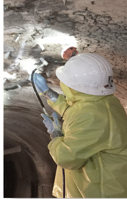
Over Head Injection with Button Head Packers
